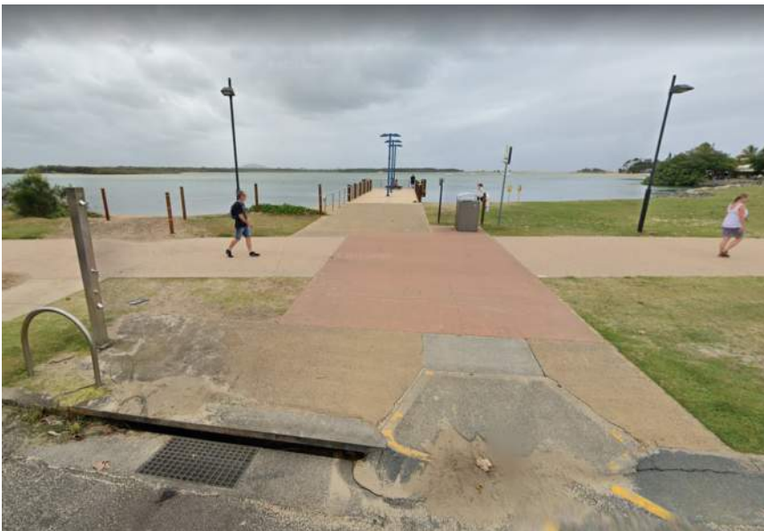
Figure 18: Existing footpath from carpark to eastern jetty. This image also shows the existing stormwater kerb drain
