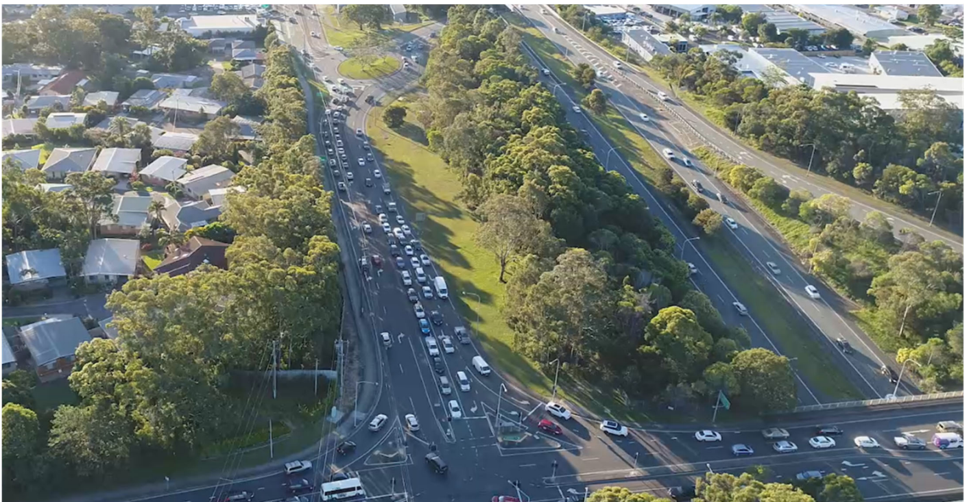
Figure 1 Large roads and intersections can divide communities and reduce the safety and attractiveness of places for pedestrians
