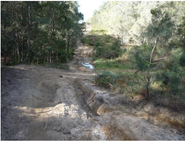
Figure 25: Eroded vehicle tracks due to unlawful off-road vehicle use along powerline in the reserve.
