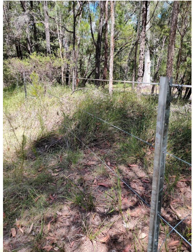
Figure 8: Fauna friendly fence installed at Brannocks Environment Reserve.
