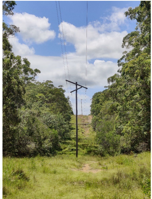
Figure 26: Power line and easement within the reserve.
