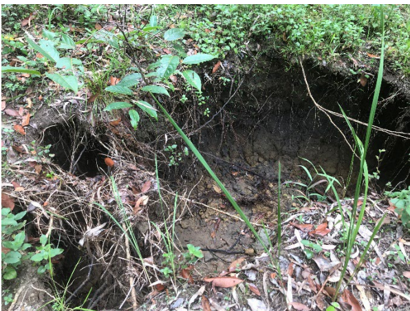
Figure 23: Evidence of sinkholes that form after heavy rainfalls.
