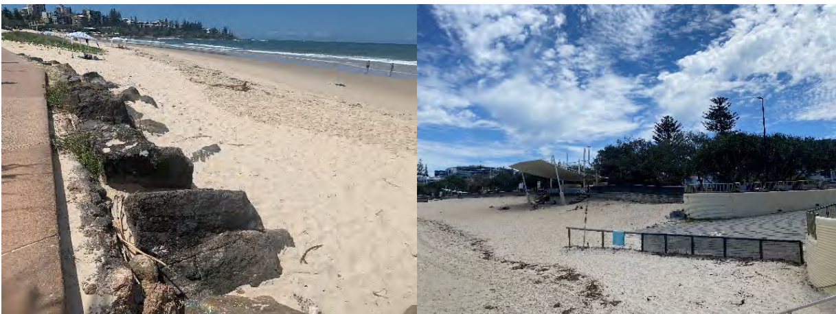
Figure 33-4: Left: Exposed footpath foundation. Right: Beach access ramp (JBP 2023)
