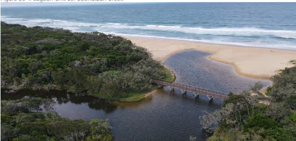
Figure 25-2: Drone image of Coondibah Creek mouth (JBP 2023)
