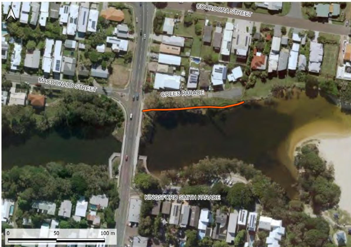
Figure 28-3: Extent of Crees Parade revetment (Unit L5, sub-unit B)
