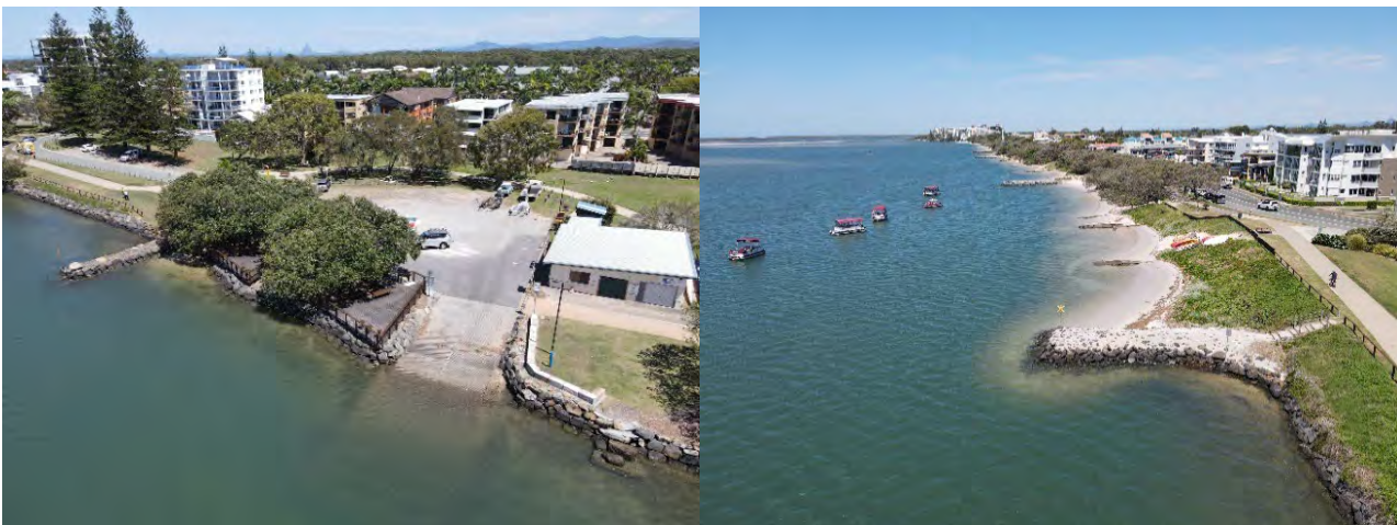
Figure 36-2: Estuary Unit E4 boat ramp, vertical seawall, and groyne structures (JBP 2023)
