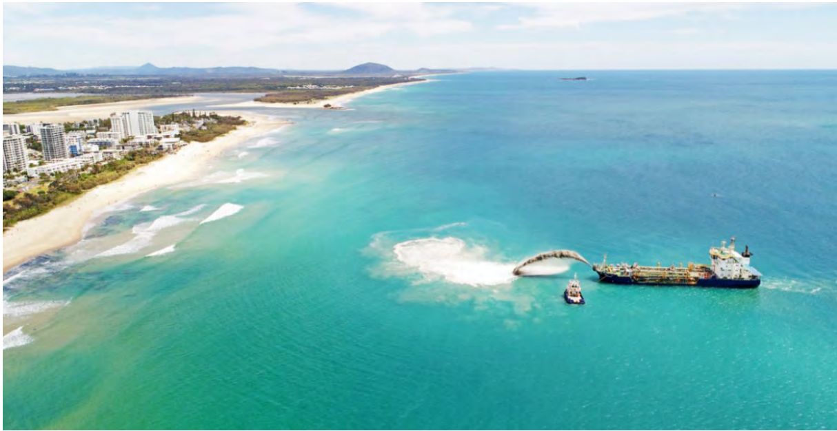
Figure 4-8: Sand being rainbowed out of the dredge during the Maroochyshore Nearshore Nourishment Trial (SCC, 2022) 16
