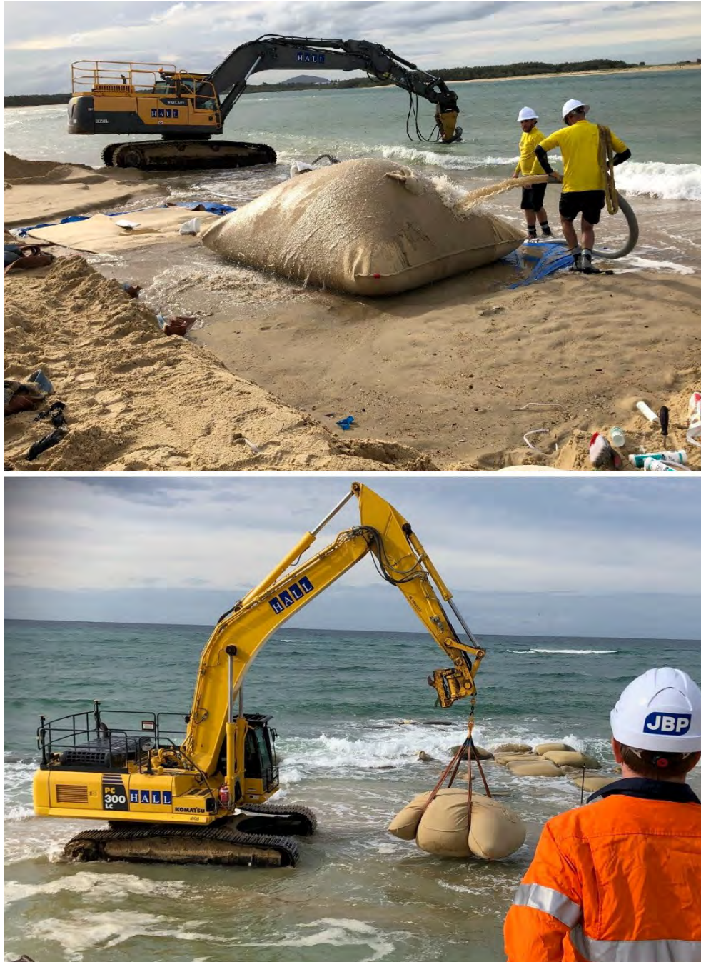
Figure 4-5: Maroochy Groynes - 8t GSC unit filling and lifting procedure (JBP 2021)
