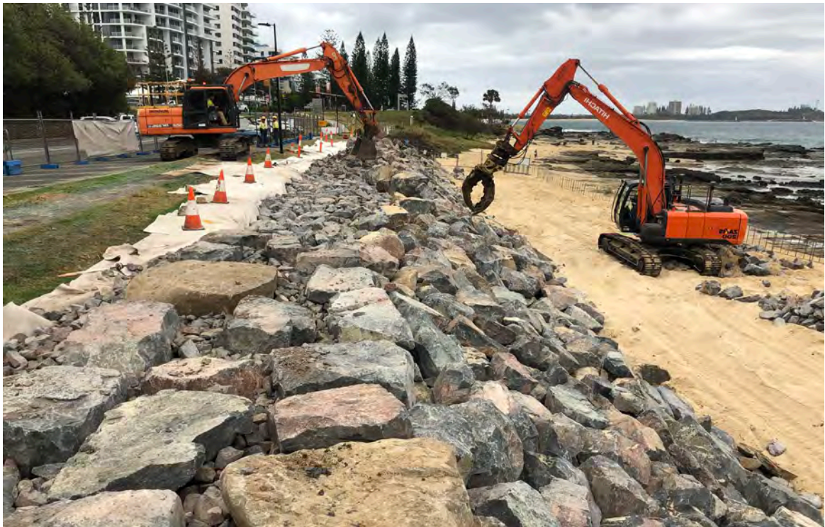
Figure 4-6: Mooloolaba Foreshore seawall during construction
